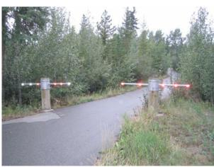
Other controls may be required to prevent vehicles from circumventing the T-bollards. Simple controls such as boulders, wood bollards, or rail fencing can be a cost effective solution.
